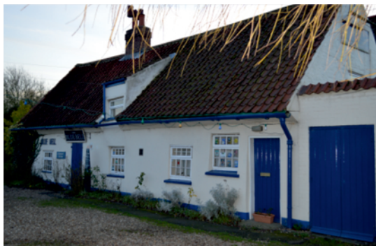
Gabled roof with later raking dormer window
