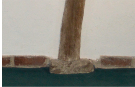
Padstone supporting post, with brick underbuilding. © Richard Croft
