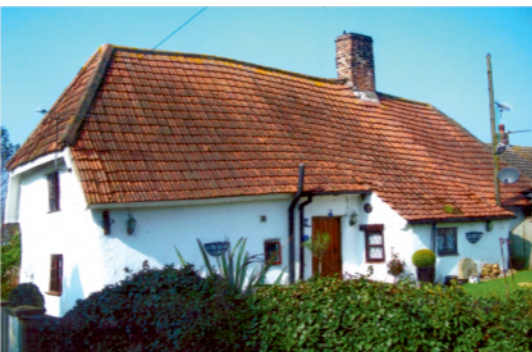
Half-hipped roof and axial stack with small outshut © Rodney Cousins
