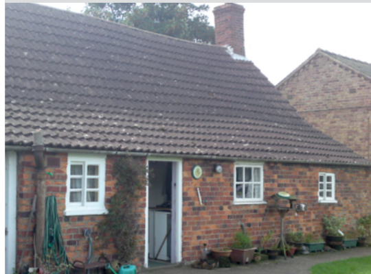
Gabled roof with catslide outshut
