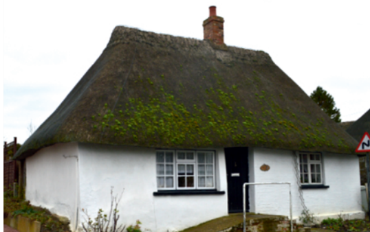
Hipped roof with axial stack
