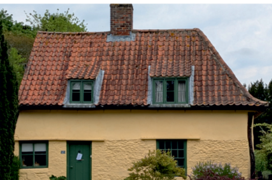
Mud and stud underbuilt in stone
