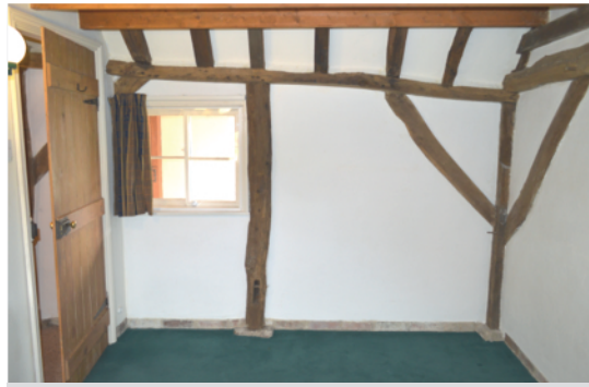
Exposed internal frame
