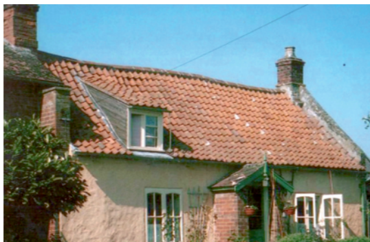
Gabled roof with gable stacks and raking dormer © Rodney Cousins
