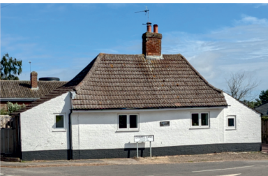
Tall chimney on a roof with tiles over thatch
