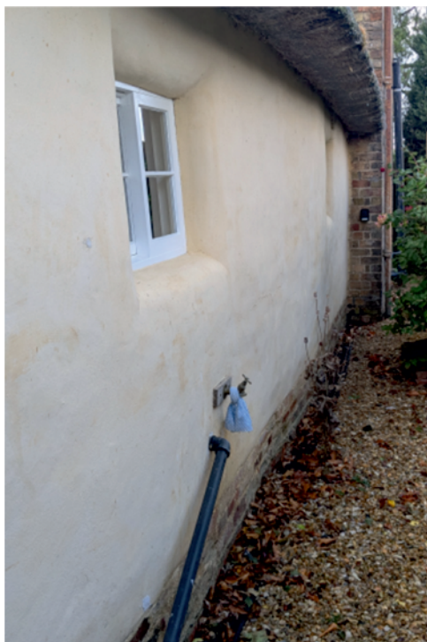
'Battered' wall tapering up
