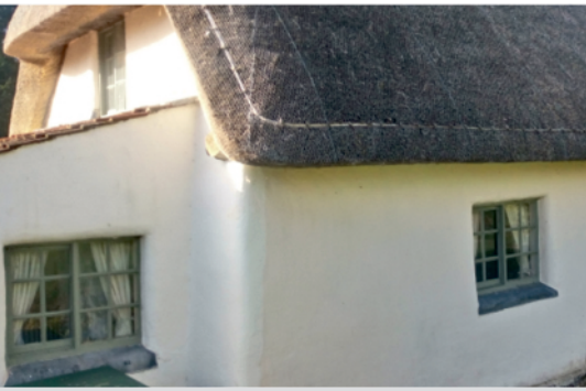
Rounded corners in thatch and daub
