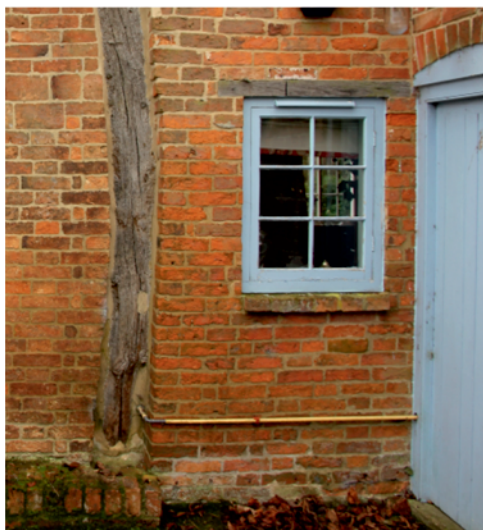
Daub replaced by brick with exposed post © Richard Croft
