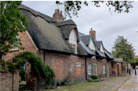
Encased mud and stud with thatch and 'tin'-covered thatch
